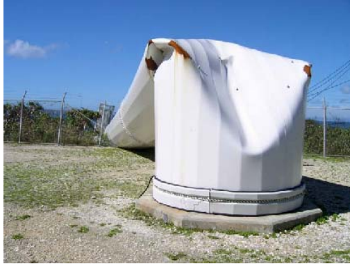
Example of collapse of wind turbine
