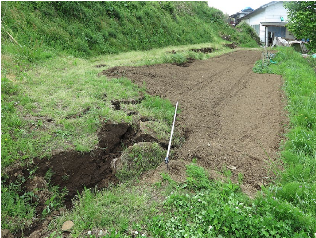
Figure 2 Surface rupture at Shimojin (N32.49519° E 130.84871°)
